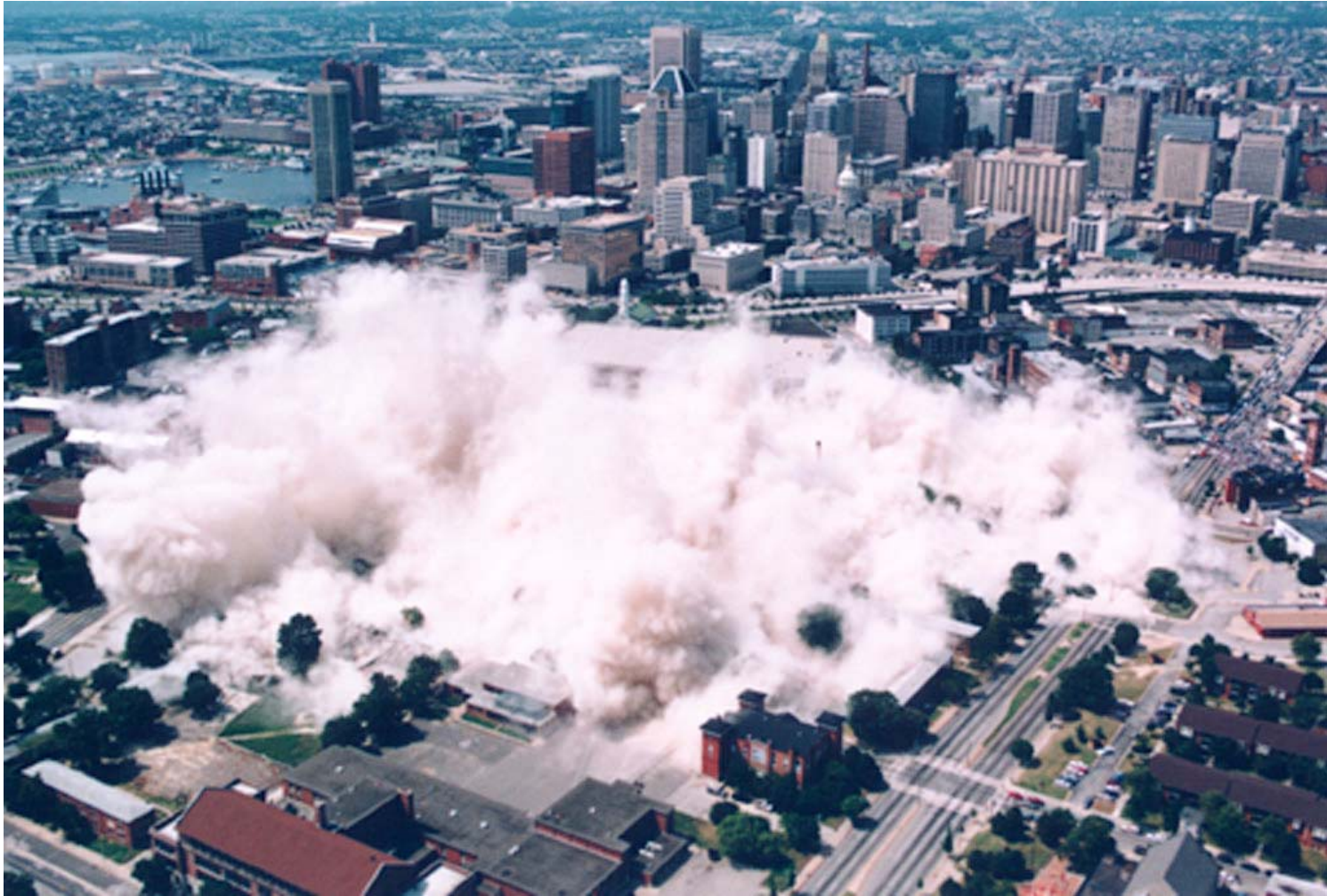
Lafayette Courts, Baltimore
