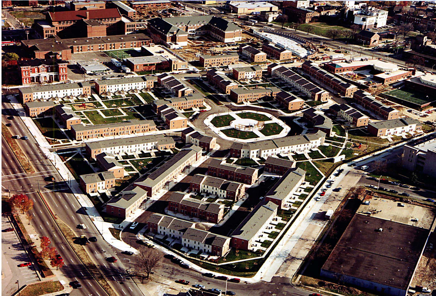
Lafayette Courts, Baltimore
