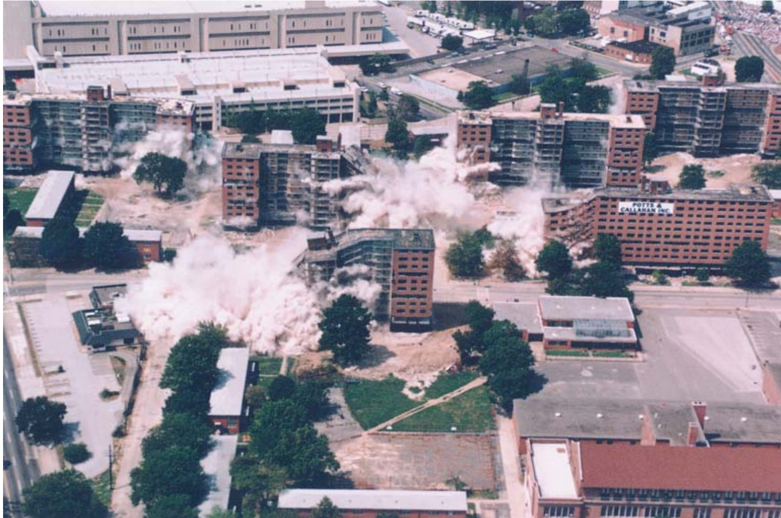
Lafayette Courts, Baltimore
